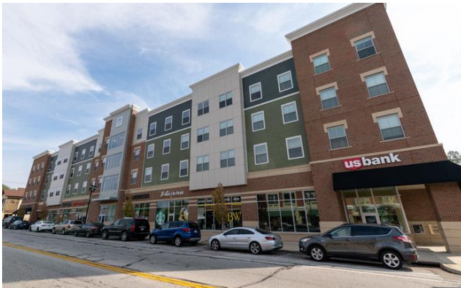
Front Street Residence Hall
