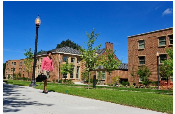
Davidson Commons Residence Hall
